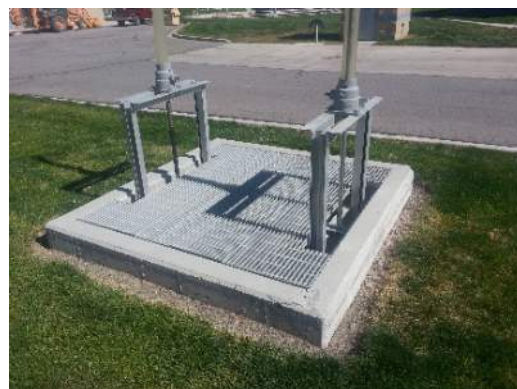
Figure 3-4 Splitter Box
