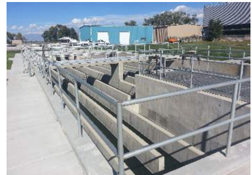
Figure 3-17 Chlorine Contact Basin
